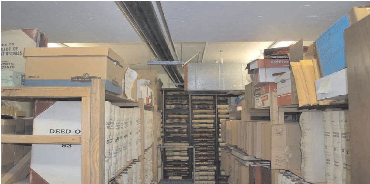
PHOTO 52: Middle aisle of basement shelving with A/C lines and water lines running through the storage area.
