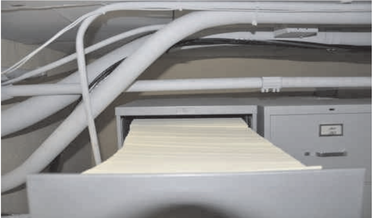
PHOTO 55: Electrical conduit located directly above filing cabinet containing Republic of Texas case files. The District Clerk is concerned about this condition.
